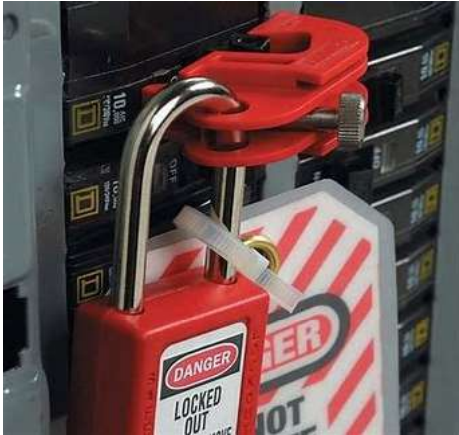
Figure 6. Breaker Lockout
