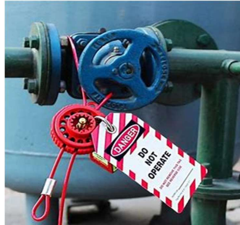
Figure 7. Valve Lockout
