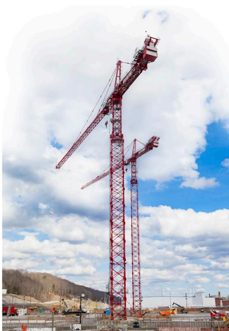
Two tower cranes, which are 300 and 360 feet tall, were installed in early 2018 as part of the construction of UPF. Having high-capacity, stationary cranes within the footprint of the buildings gives UPF the ability to reach every spot in the construction zone, making materials handling safe and efficient.
