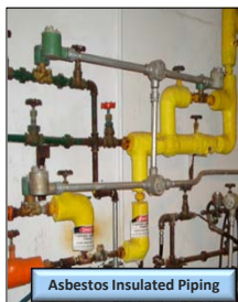
Asbestos Insulated Piping
