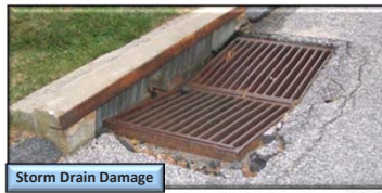
Storm Drain Damage
