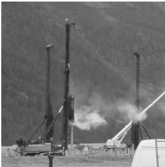
Figure 1: Friction-caused ignition of cushion block
