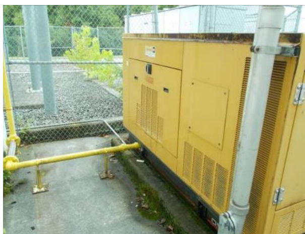
Figure 3-27. Emergency Generator
