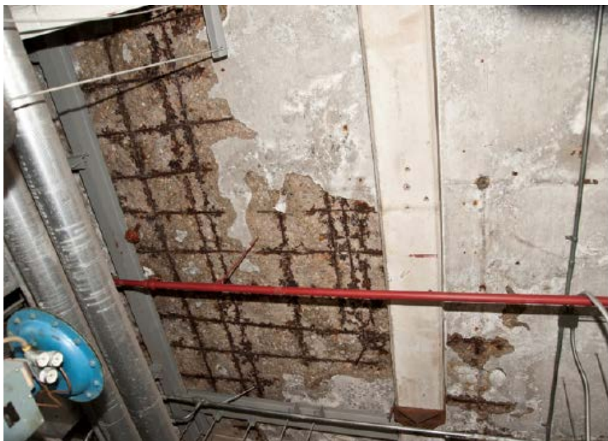
Figure 1-6. Spalling Ceiling of Fan Room 1
