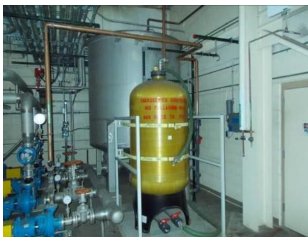
Figure 3-29. Indoor Aboveground Storage Tanks
