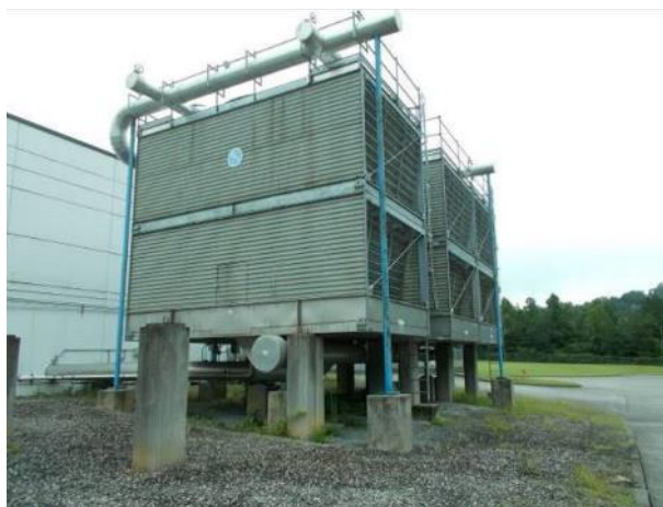
Figure 3-25. Cooling Towers
