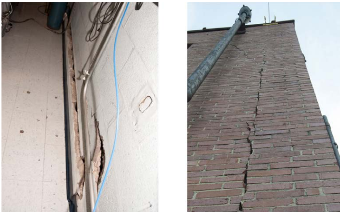
Figure 1-4. Bulging Wall in Room 270 of Building 9202 (left) and Cracked Brick Façade on the West Wall of Building 9202 (right)
