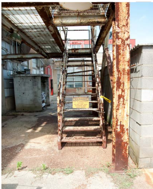
Figure 1-7. Unsafe and Unusable Emergency Stairs
