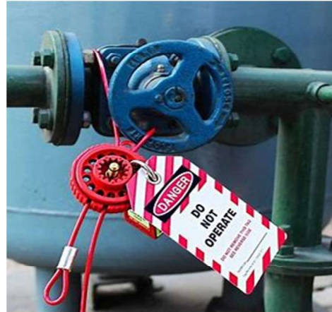
Figure 7. Valve Lockout
